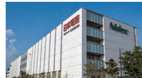
Nidec Research and Development Center, Japan Operates Entirely on Renewable Energies
