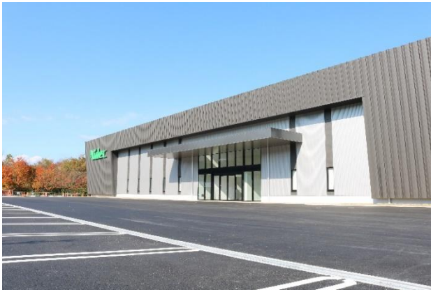
Exterior of the new technical center
